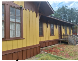
Lindsborg Union Pacific Train Depot (1879-1972) -New exterior paint
